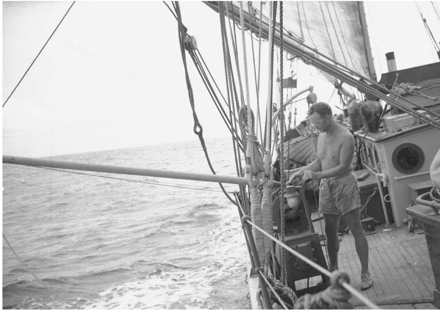
Figure 2. Scientists used the bathythermograph, or BT, shown here on deck, to measure temperature and to identify the depth of any sharp changes that might obstruct the efficacy of sonar. (Courtesy of Woods Hole Oceanographic Institution.)
